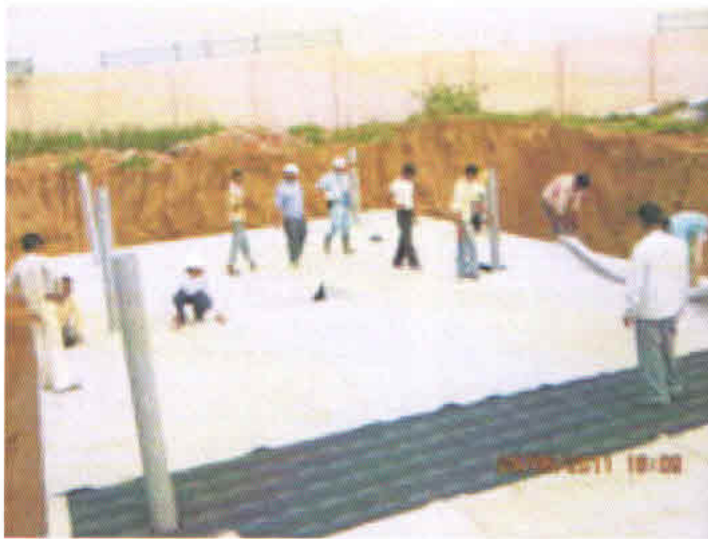
Picture 1: Showing installation of modular tanks at Honda Scooters and Motorcycles In Tapukra, Rajasthan and Bangaluru and Metro Rail Delhi.
